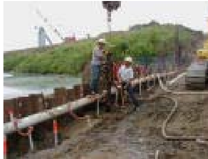
Pumping in progress
